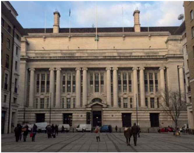
The view of the entrance across Forum Magnum Square
